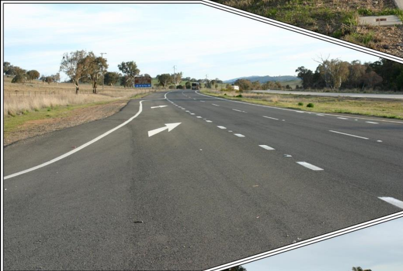
Plate 5.9: Left turn acceleration lane for southbound departure lanes of Hume Highway from Paynes Road (Ref: E724-A084)
