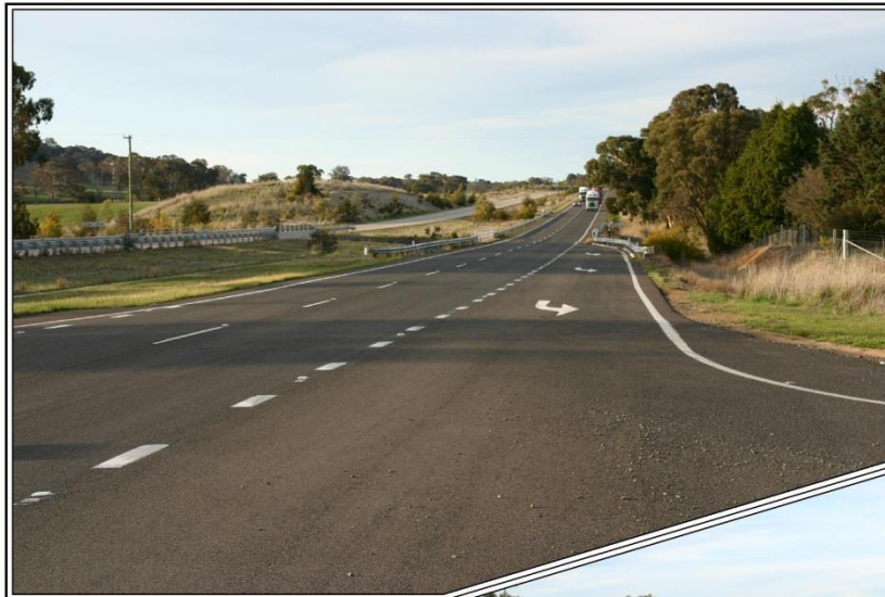
Plate 5.7: Left turn deceleration lane from the Hume Highway into Paynes Road (Ref: E724-A083)
