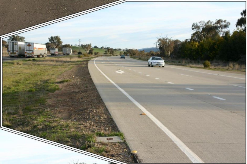
Plate 5.8: Right turn bay within the northbound lanes of the Hume Highway into Paynes Road (Ref: E724-A085)
